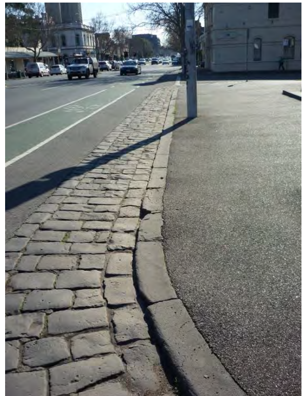
Figure 7 Contributing to significance within the heritage place HO1. Bluestone kerbstones and coursed bluestone pitcher gutters. July 2015.
