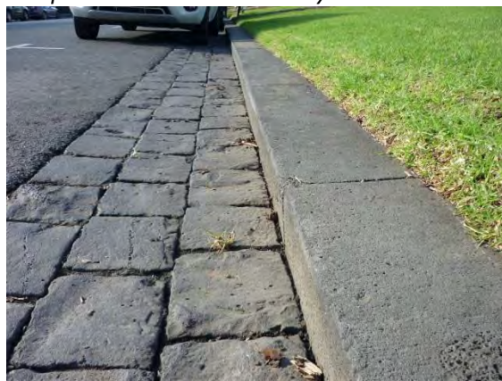
Figure 16 Kerb and coursed gutter meeting the lawn surface. July 2015
