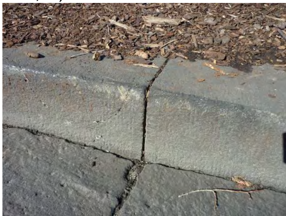
Figure 14 Fine tooling marks evident on the ashlar bluestones which form the kerb. MacArthur Place North. July 2015
