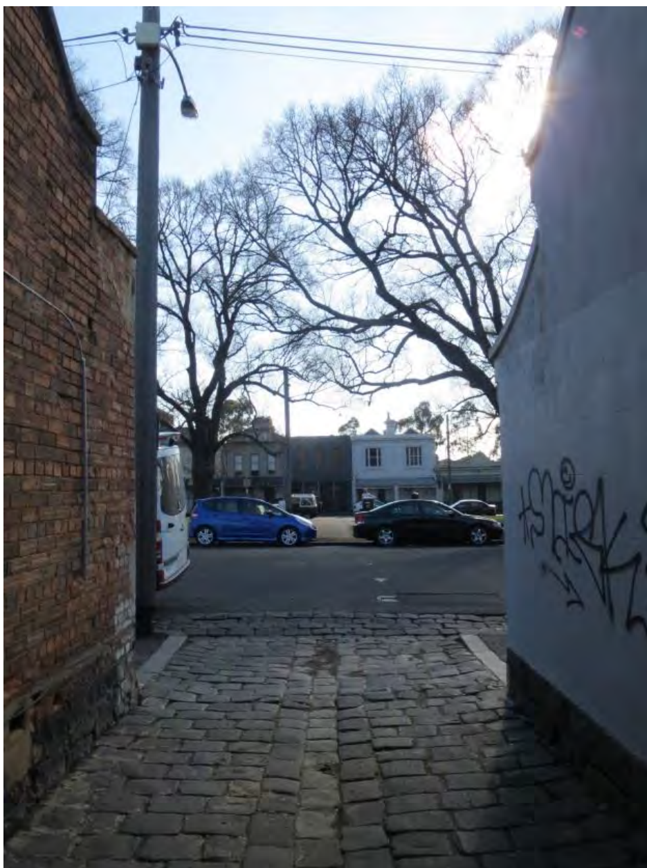
Figure 8 CL1059, looking north in alignment with the central path to the Square. Lanes surfaced with bluestone pitchers intersect with the bluestone street gutters. July 2015. Lanes, bluestone kerbs and coursed gutters, the elm tree rows and green space, and the graded perimeter buildings, all contribute to significance within the heritage place HO1. .
