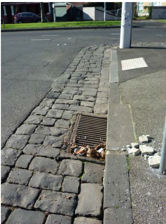
Figure 17 Bluestone kerb and coursed gutter. South east, at Canning Street intersection. July 2015.
