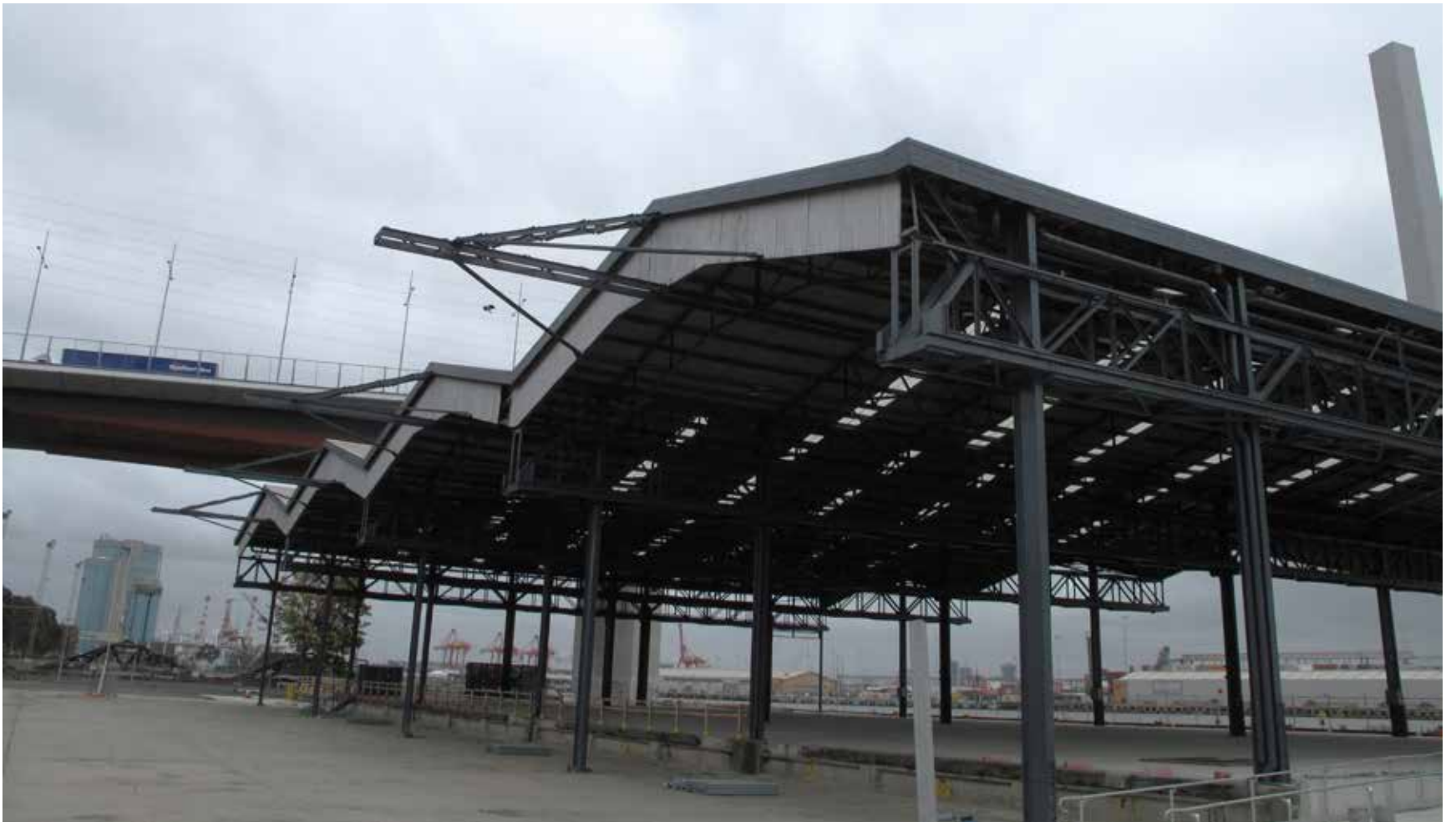
Shed 21 with the overhead crane projections visible. (City of Melbourne)
