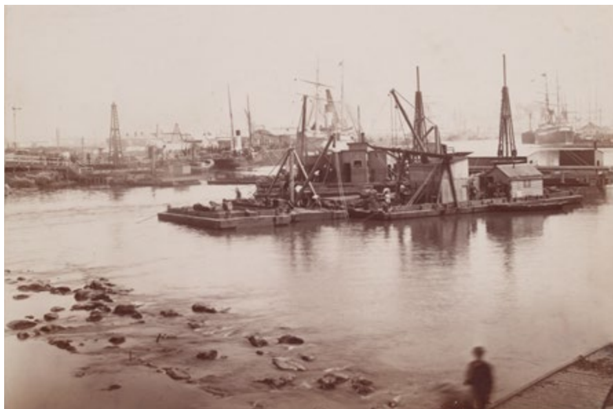
Image 6. This photograph shows the Yarra falls (the rocks in the foreground) being removed in 1883. The dredges can be seen hauling away large rocks.
