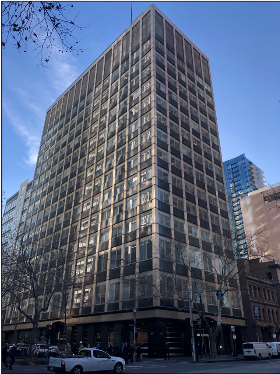
Figure 6 The former Reserve Bank of Australia to the corner of Collins and Exhibition streets. The original pale marble of the ground floor columns that rose through the height of the building has been replaced or overclad with segmented steel cladding. A cornice at the summit of the building replaces the original spandrel panels and further changes the language of the building. At the ground floor, another cornice treatment establishes a visual break between the ground and first floors.
