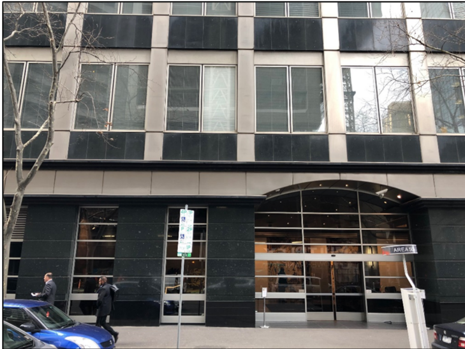
Figure 7 Image showing the west elevation of the RBA building to Exhibition Street. The non-original segmented stainless steel cladding to the columns of the upper levels, granite clad piers and infill glazing of the ground floor level are apparent.
