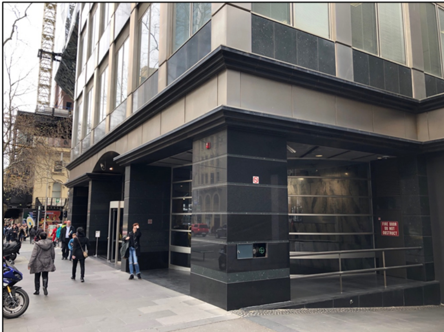
Figure 8 The non-original (wide) piers, cornices and curved glazed wall to Collins Street.
