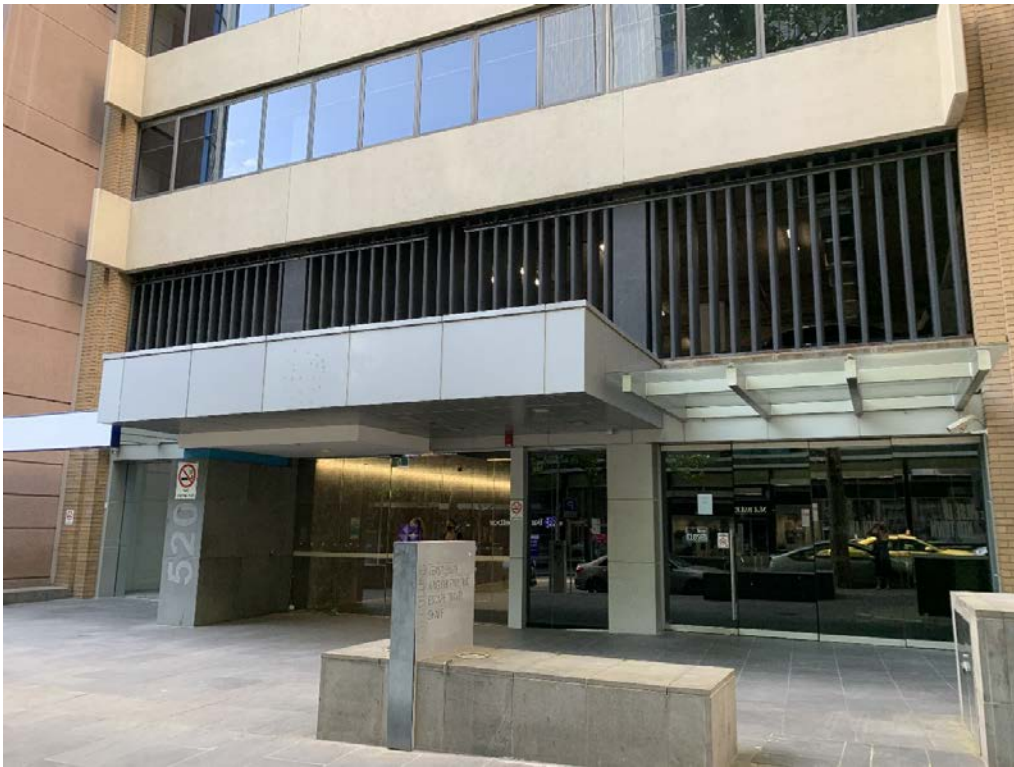
Figure 3-16 View of the modified forecourt to Collins Street, altered ground floor level and painted concrete fins to the carpark above
