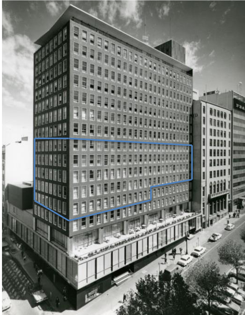
Above: The area enclosed with the blue line has had its steel frame sash windows shown here removed and replaced with fixed glazed panels.
