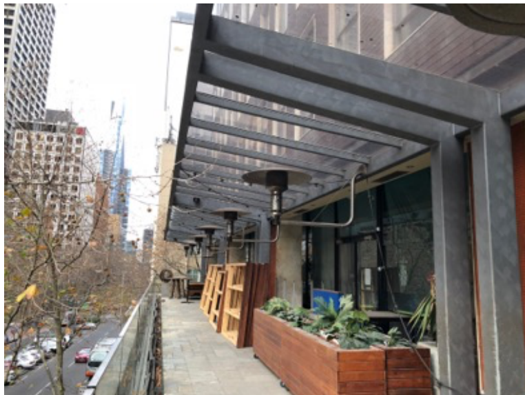
Above: Balcony today, with steel frame glazed awning fitted and new frameless glazed balustrade.
