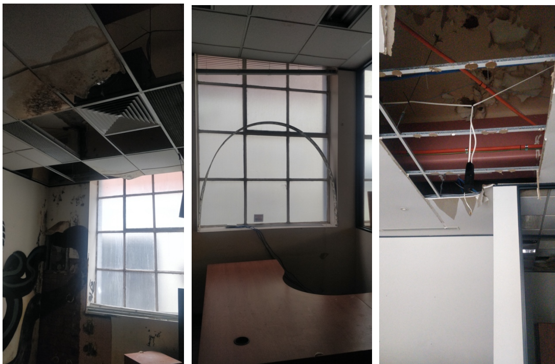
Figure 6: Internal views showing original steel-framed windows and general water damage to walls and ceilings. Source: Trethowan Architecture, 2021.
