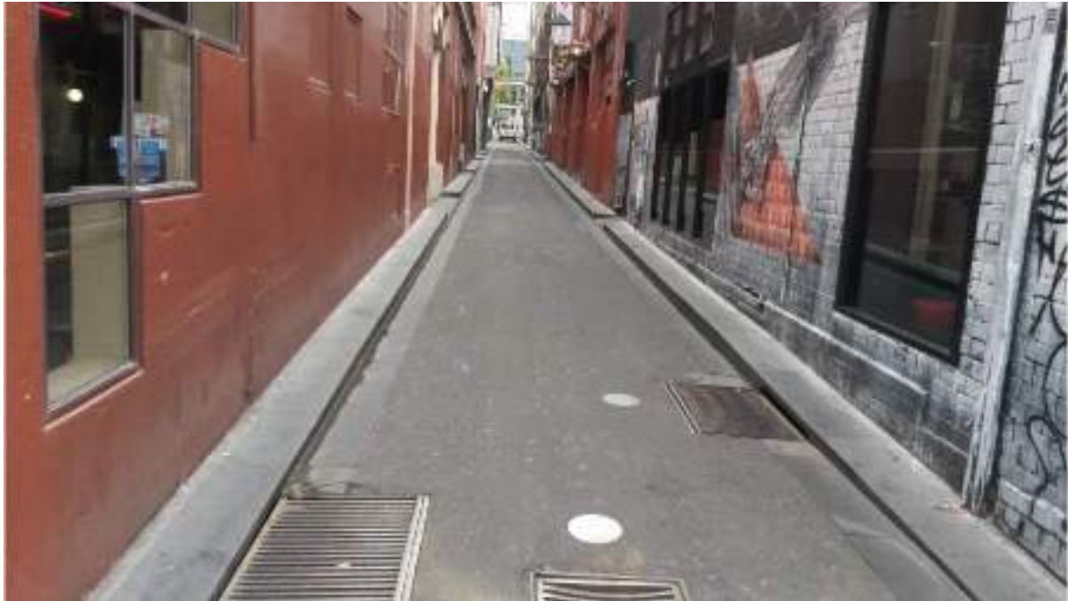
Figure 0-3 Typical grated kerb pits and lane-type pits
