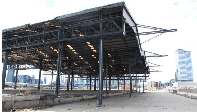
The south side of Shed 21 with the trays that held the electrical supply for the transverse cranes which extend over the truck loading bay. The extent recommended in the In-depth Heritage Review 2021 includes the roadway to the right of the photograph up to the fence. (P Mills 2019)
