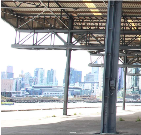
Figure 7: The flat, parallel chord trusses originally extended past the building towards the river and were supported on columns but have now been cut off. They supported the seven bridge cranes which have been removed. The reinforced extension of the columns can be seen near the base. (P Mills, 03/04/2018)
