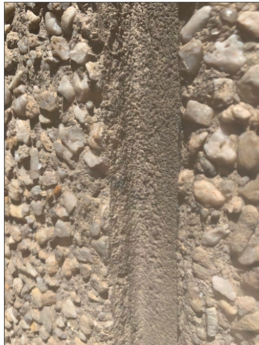
Figure 6 Detail of the aggregate concrete panelling of north and west facades.
