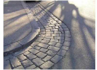
A traditional bluestone kerb and pitcher channel in North Melbourne. These add to the neighbourhood's character and heritage significance and should be conserved through timely maintenance and careful repairs when necessary that match the existing details.
