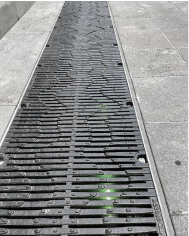
Custom grates designed to reduce litter entering waterways
