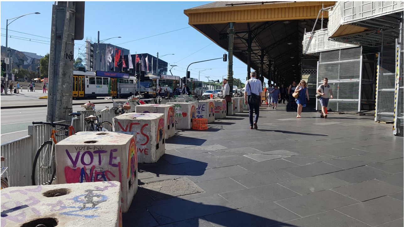
Figure 12: Concrete bollards installed across Hoddle Grid to prevent hostile vehicle attacks (photo taken at the corner of Flinders Street and Swanston Street, outside Flinders Street Station)
