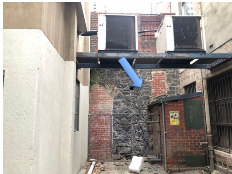
The south elevation of the rear addition to 287-289 Elizabeth Street, viewed from Mitchell Lane. The wall contains remnants of the bluestone wall of an earlier building (marked with an arrow).
