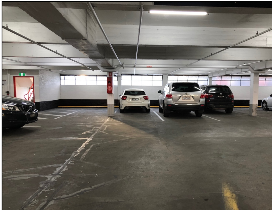
Figure 16 Interior view looking east at the first floor of the car park showing the open plan form behind the Warburton Lane elevation and the exposed concrete structural system.
