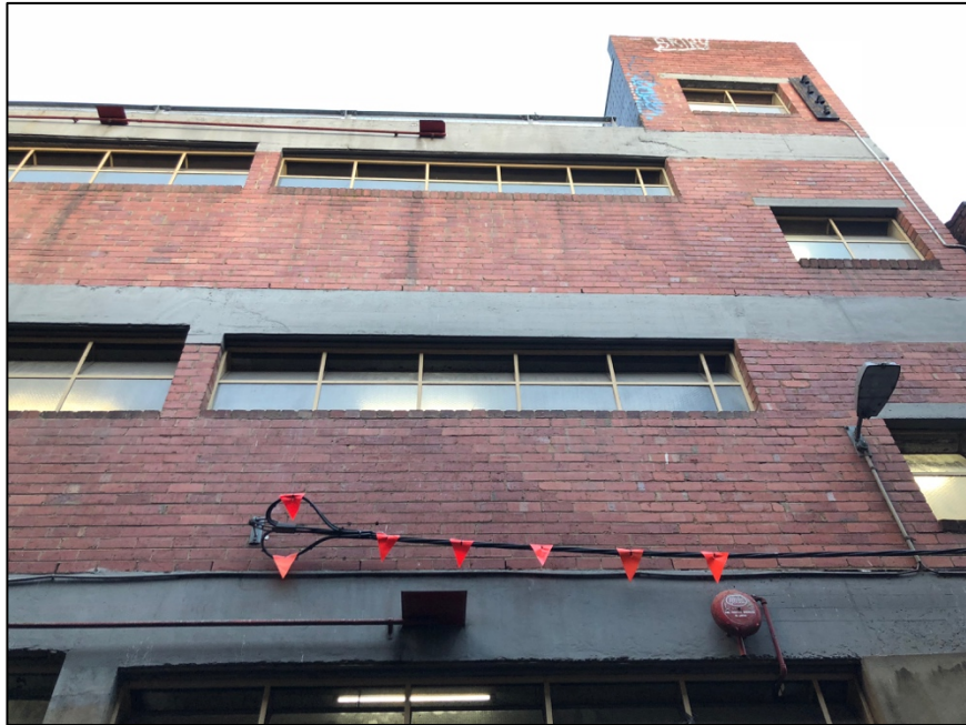
Figure 13 View of the upper levels of the Warburton Lane elevation of the subject site showing the metal framed windows and concrete structural banding.
