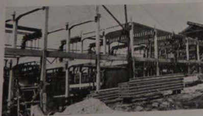
General view of new building erected for William Angliss and Co. (Aust.) Pty. Ltd. at Footscray, Victoria. Precast concrete structural members are clearly shown.
