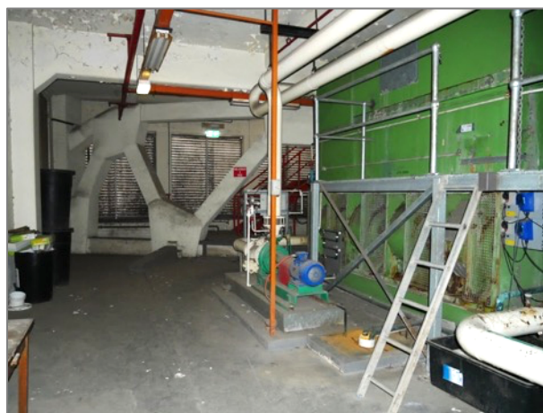
Figure 37. Interior of first floor (now plant room) showing the structure added to support building (May 2018)
