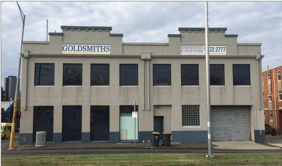
Figure 10. The northwest elevation fronting Hawke Street, which was originally composed of two symmetrical elevations each with a central entrance but is no longer evident in the openings to the ground floor.
