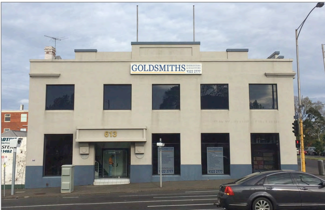
Figure 9. The northeast elevation fronting King Street with a modern stepped pediment and modern entry canopy with oversized corbel brackets.
