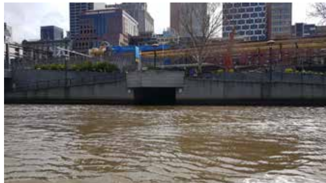
Image 59. Elizabeth Street main drain outlet underneath Flinders Walk
