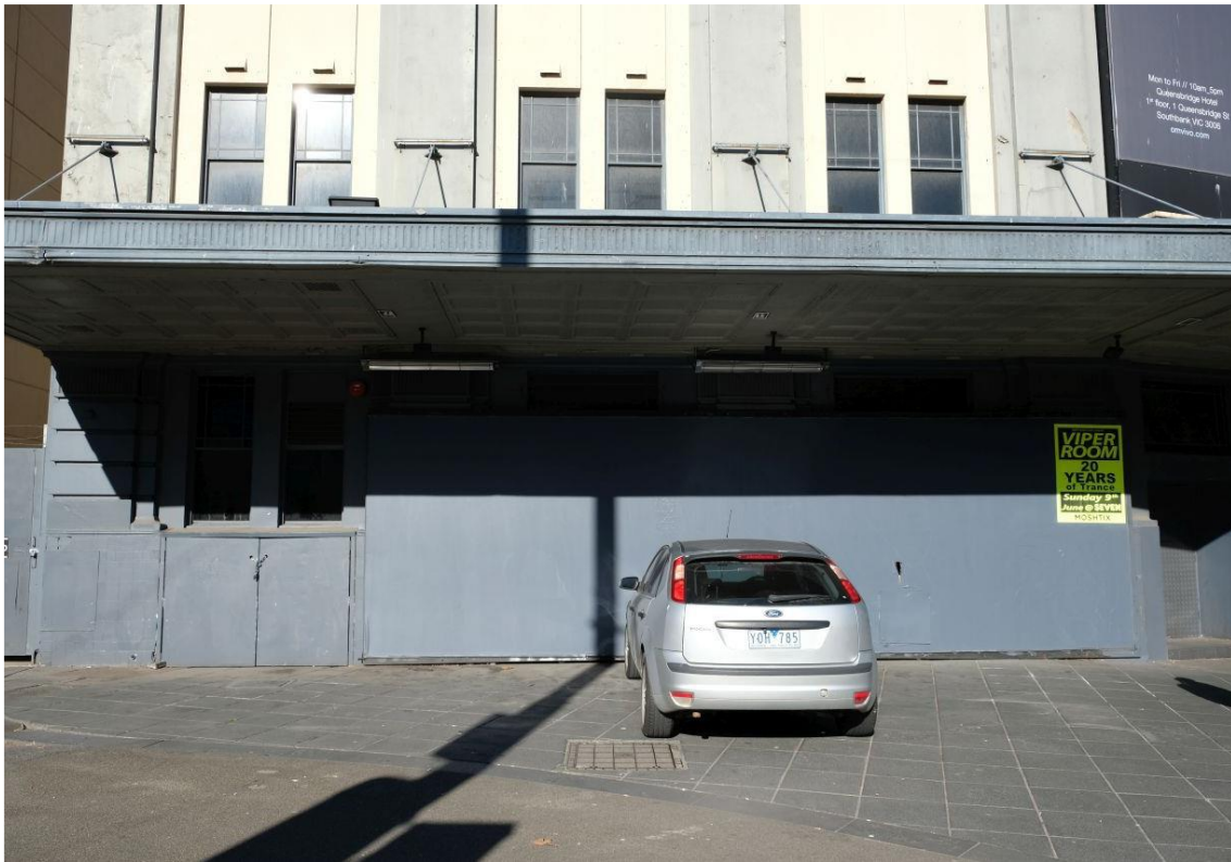
Figure 14 View of the ground level façade showing the boarding over of openings
