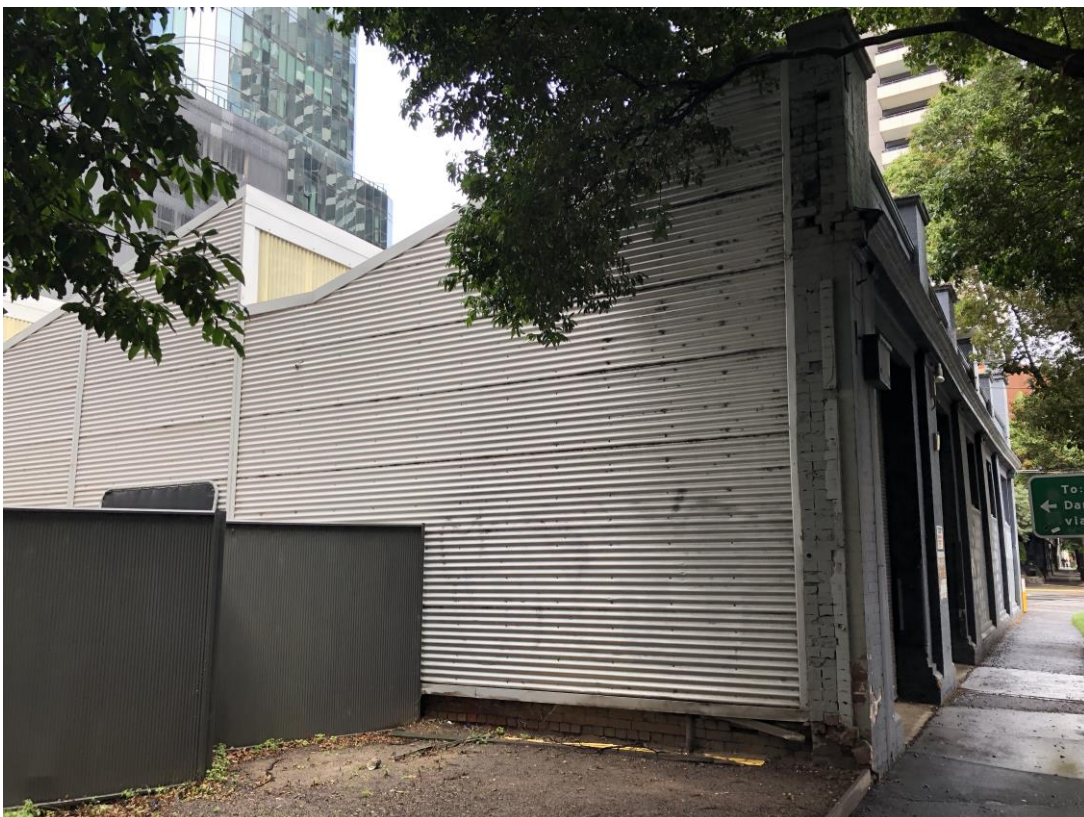
Figure 21 The east elevation on Haig Street showing the new east wall and reclad roof where the two eastern bays have been demolished
