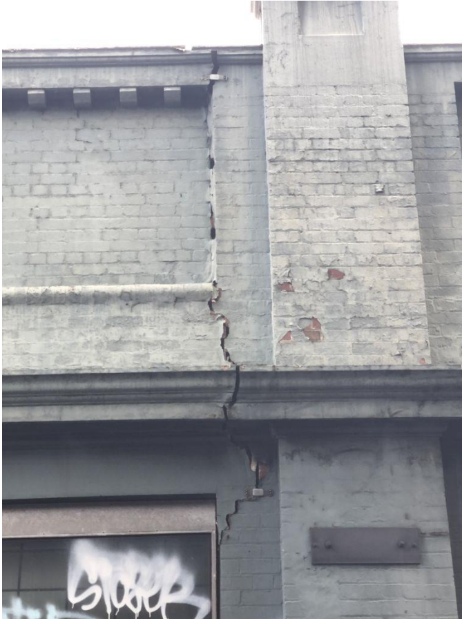
Figure 16 Major structural cracking in the return facade on Haig Lane
