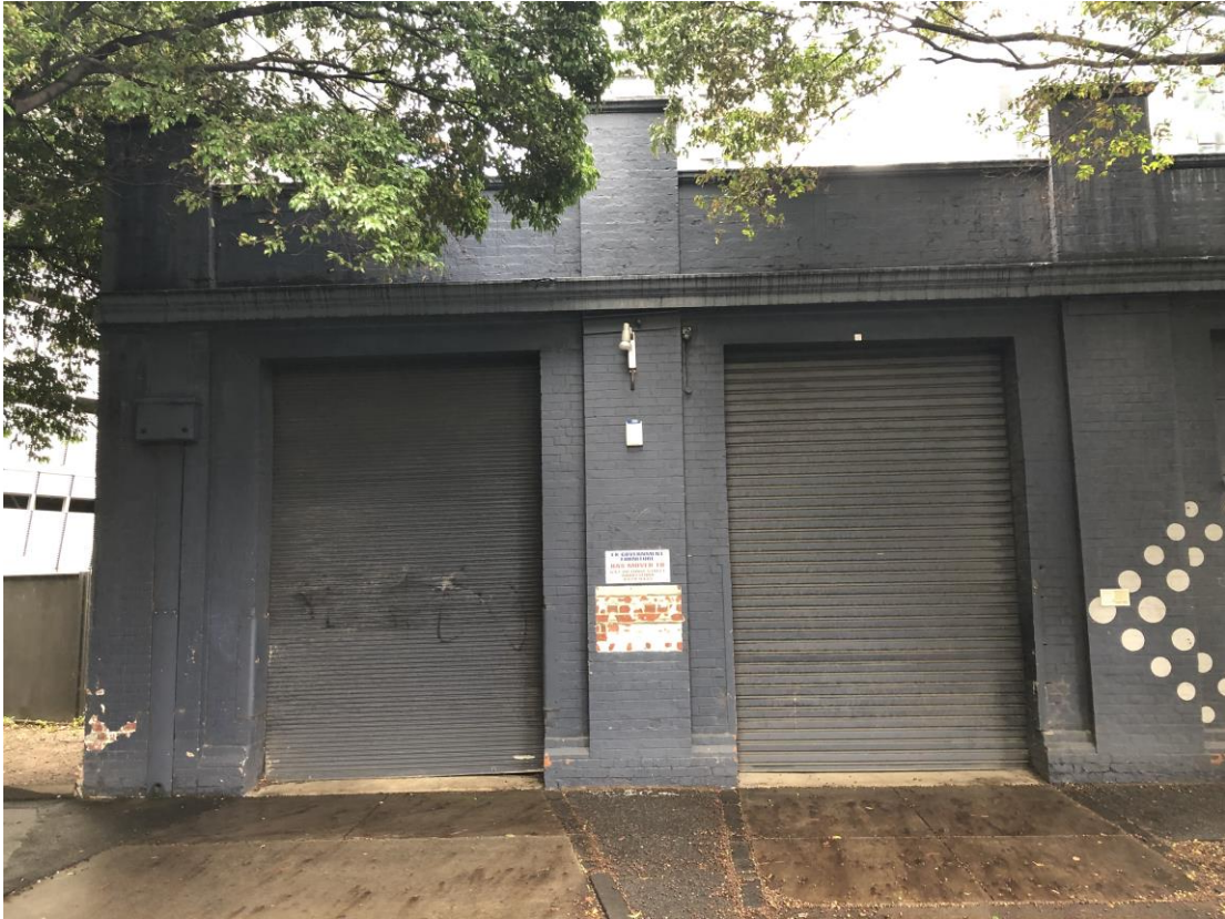
Figure 20 Vehicle openings on Haig Street; the opening to the right was originally a highlight window
