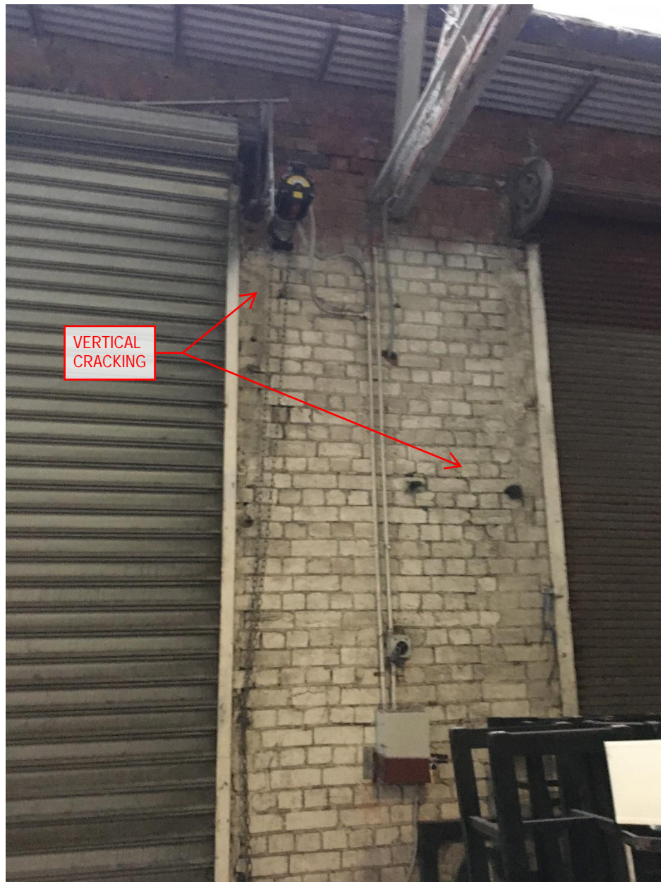
Image 2.2: Vertical cracking in masonry wall at connection to roller door rails. Horizontal cracking above roof truss connection.
