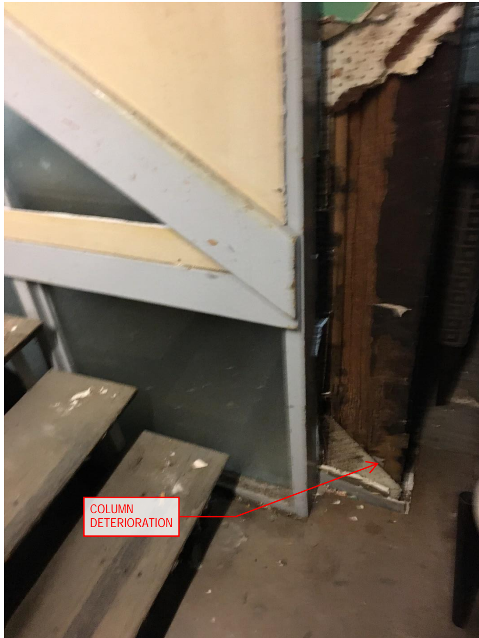
Image 2.9: The existing timber column at the base of the stairs to the first floor has significantly deteriorated. The damage requires repair in the short term.
