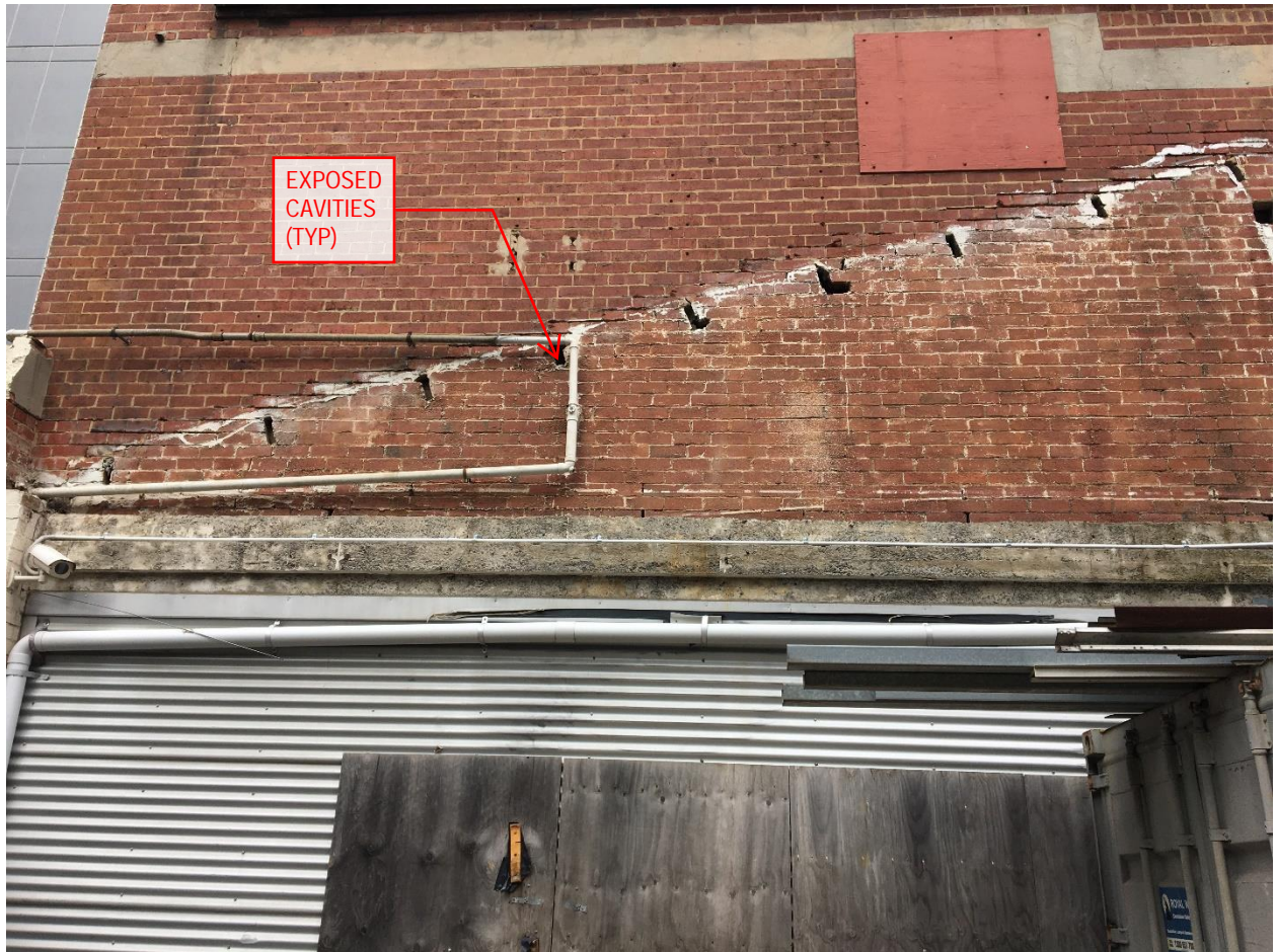
Image 2.16: Exposed cavities in masonry due to demolition of adjacent structure
