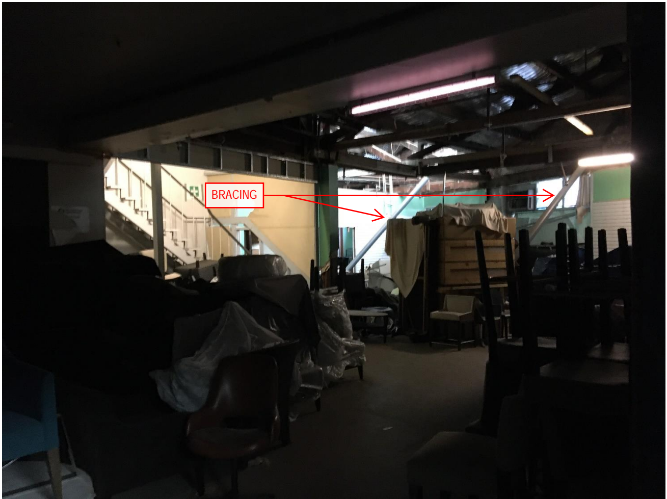
Image 1.4: Bracing of Façade at Corner of Clarendon St and Haig Lane
