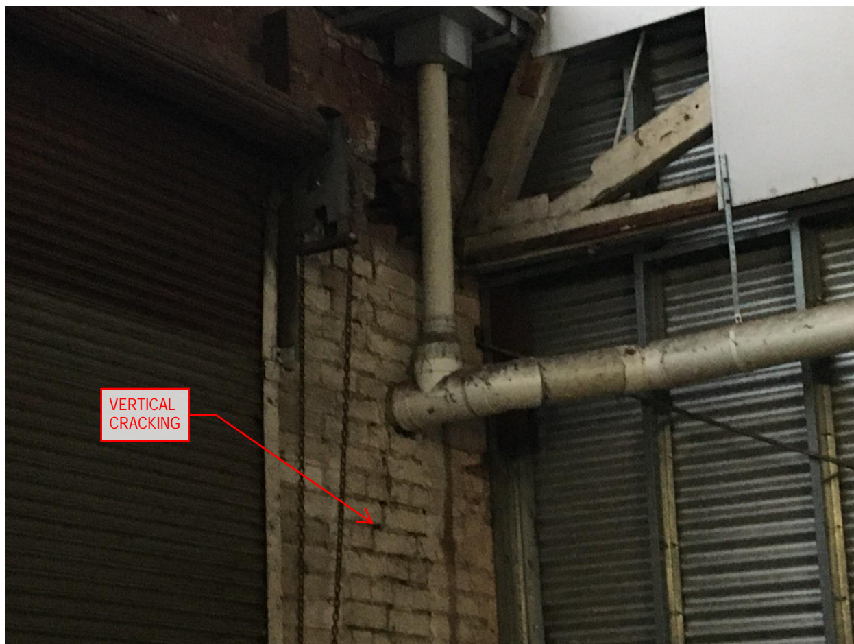
Image 2.1: Vertical cracking observed at door lintel, intersection of roof truss and downpipe.
