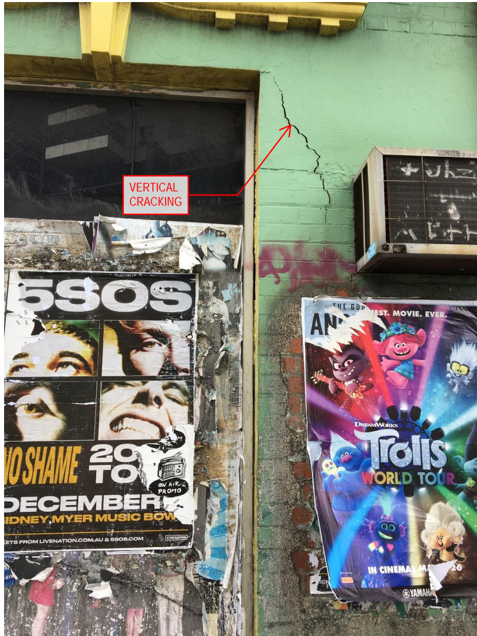
Image 2.15: Cracking in masonry and mortar joints below a lintel.
