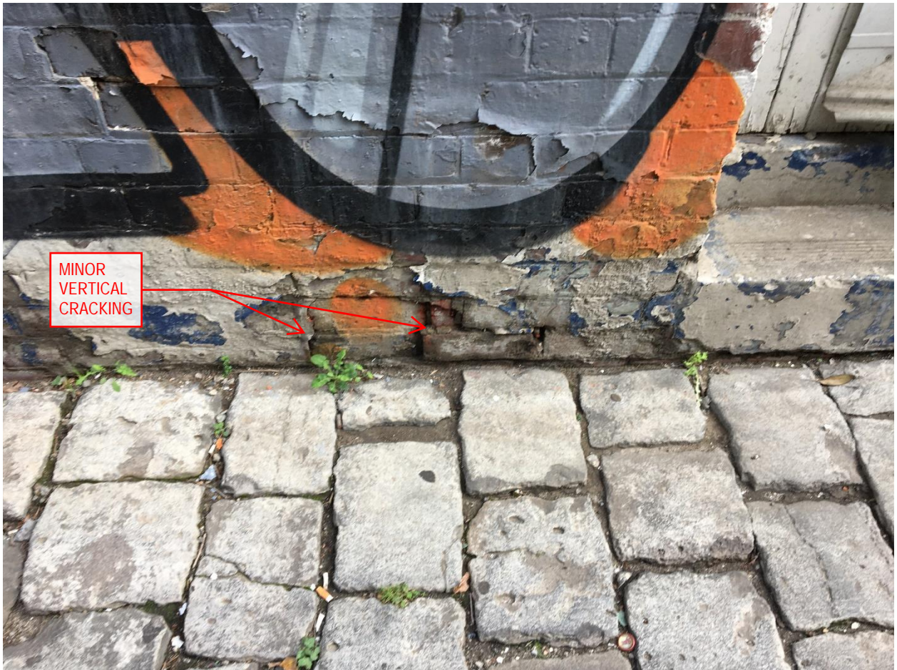
Image 2.14: Minor cracking in masonry mortar joints.
