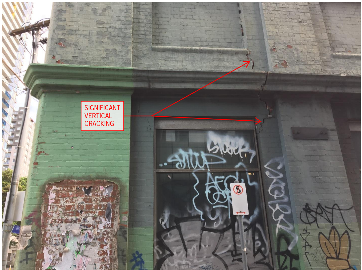
Image 2.12: Significant vertical cracking to the masonry façade. Outward lean of the wall, which is braced behind.
