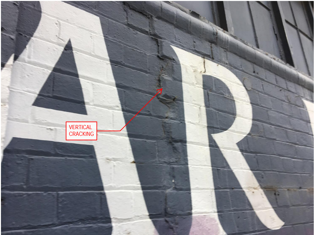
Image 2.17: Vertical cracking/step out of masonry façade.
