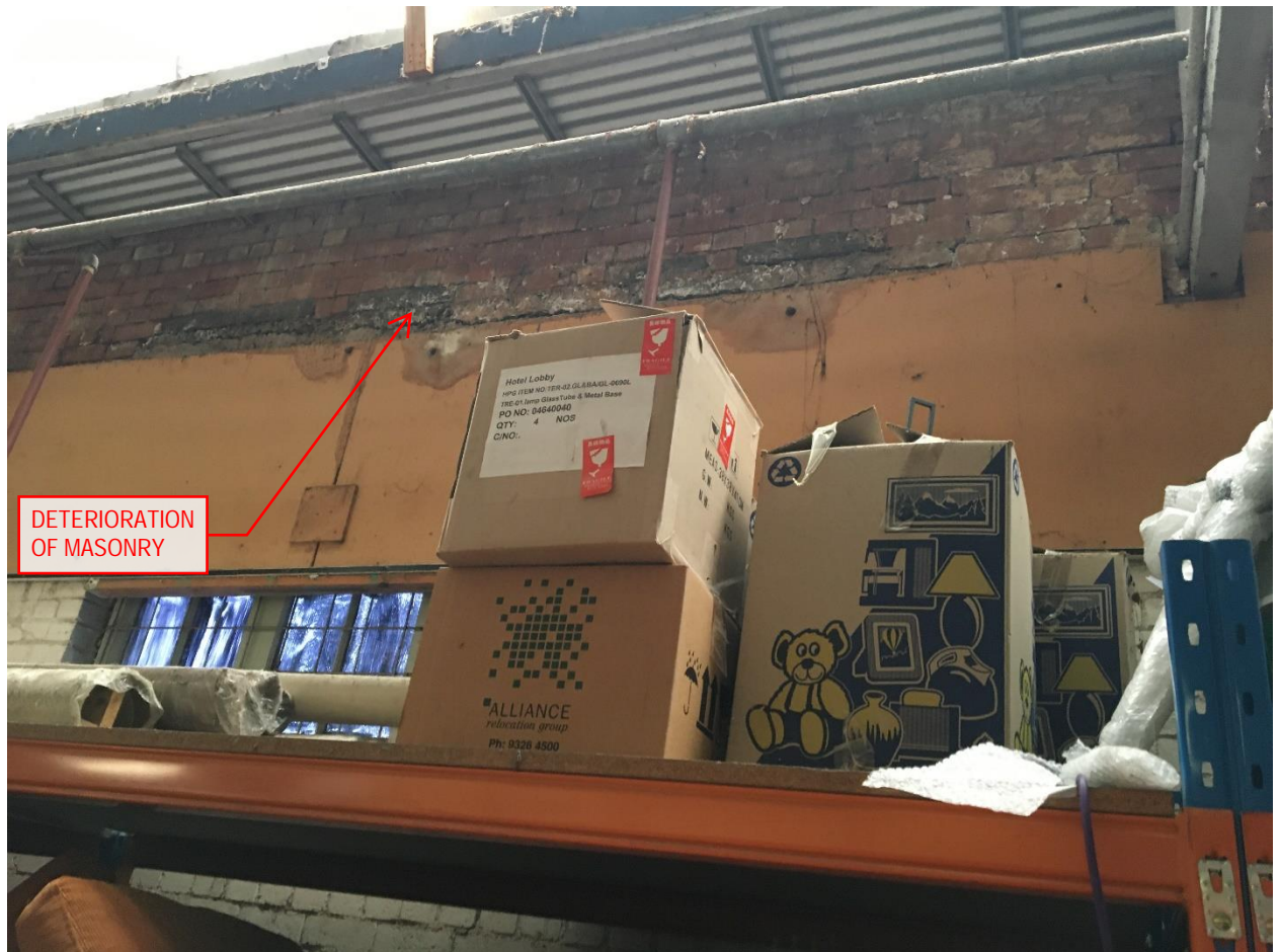
Image 2.4 Significant deterioration of existing masonry above lintels. Horizontal cracking above connection to timber truss.
