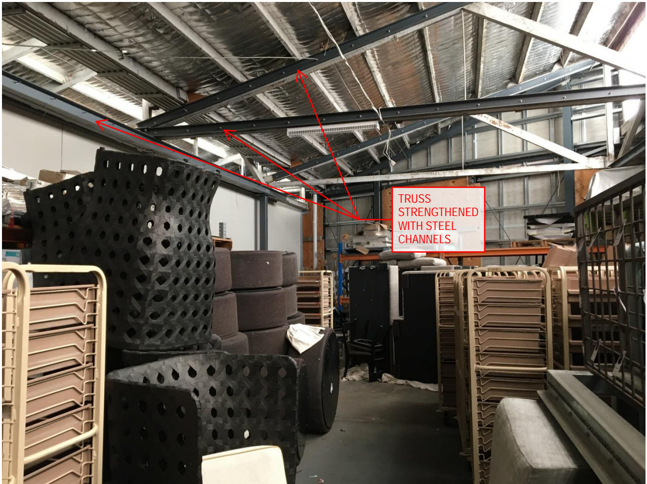
Image 1.3: Timber trusses strengthened with steel channels each side. The Clarendon St steel framed wall in the background.
