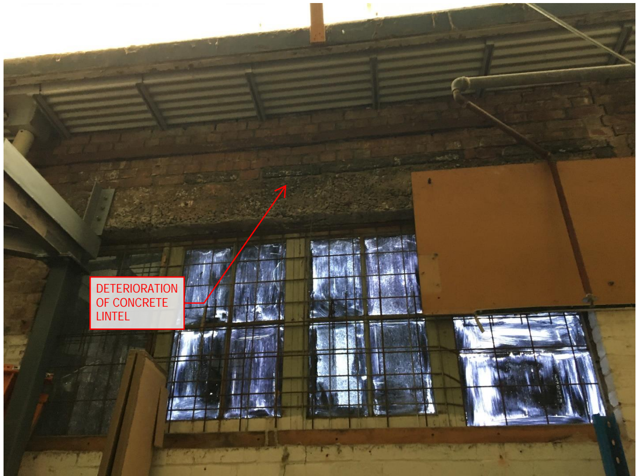
Image 2.6: Concrete lintel deterioration
