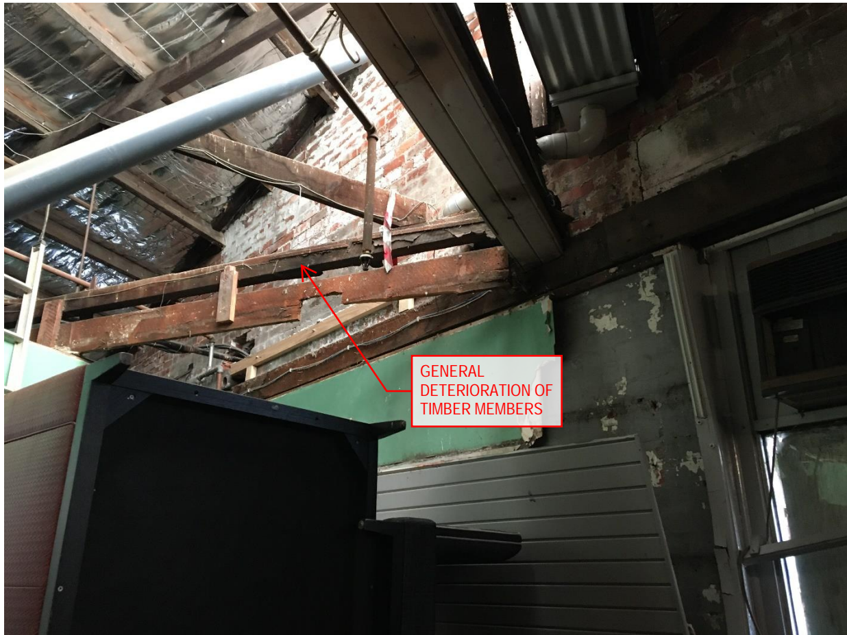
Image 2.11: Southern Store timber truss deterioration.
