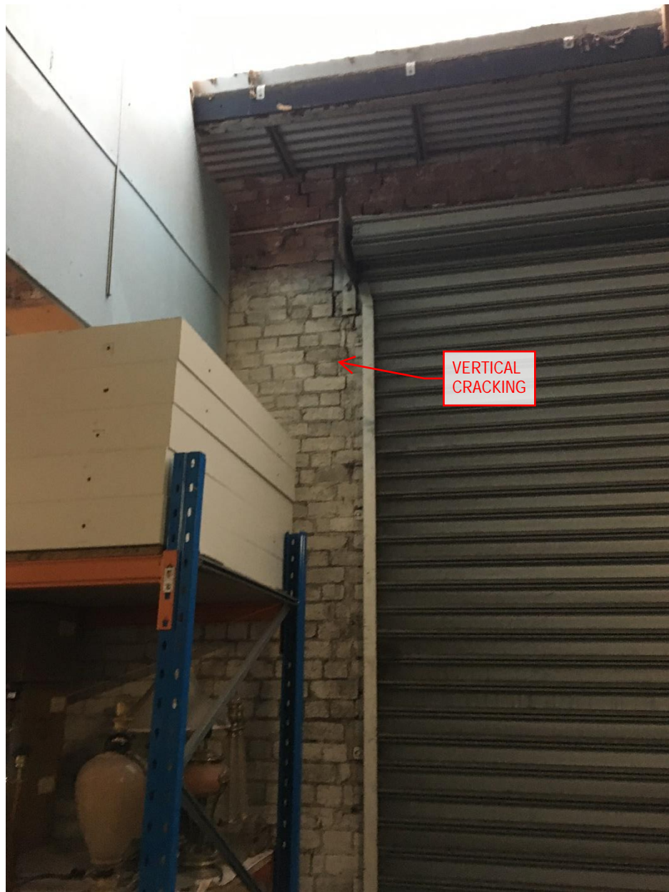
Image 2.3: Vertical cracking in masonry wall above and below connection of roller door header. Vertical cracking at connection of roller door rail.
