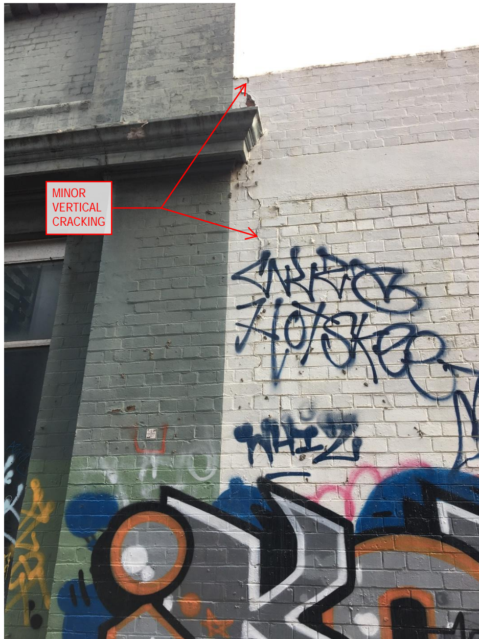
Image 2.13: Minor vertical cracking at the transition in parapet heights
