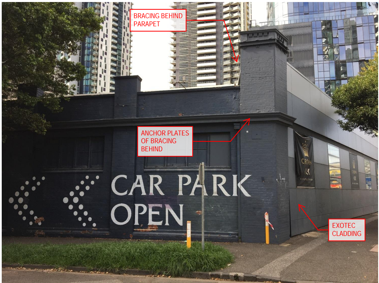
Image 1.1: Corner of Clarendon and Haig St, showing Exotec cladding on Clarendon St.
