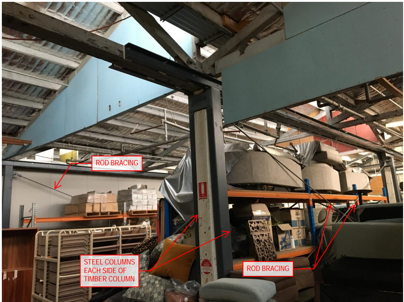
Image 1.2: Steel column strengthening of timber columns, with vertical rod bracing between columns
