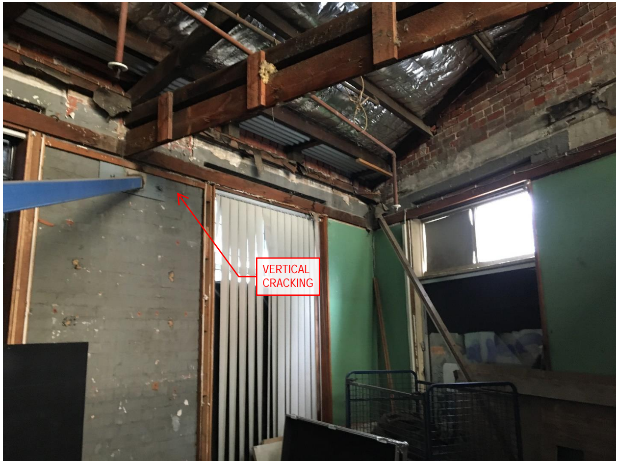
Image 2.10: Minor vertical cracking adjacent to steel brace. Internal view of item 12.
