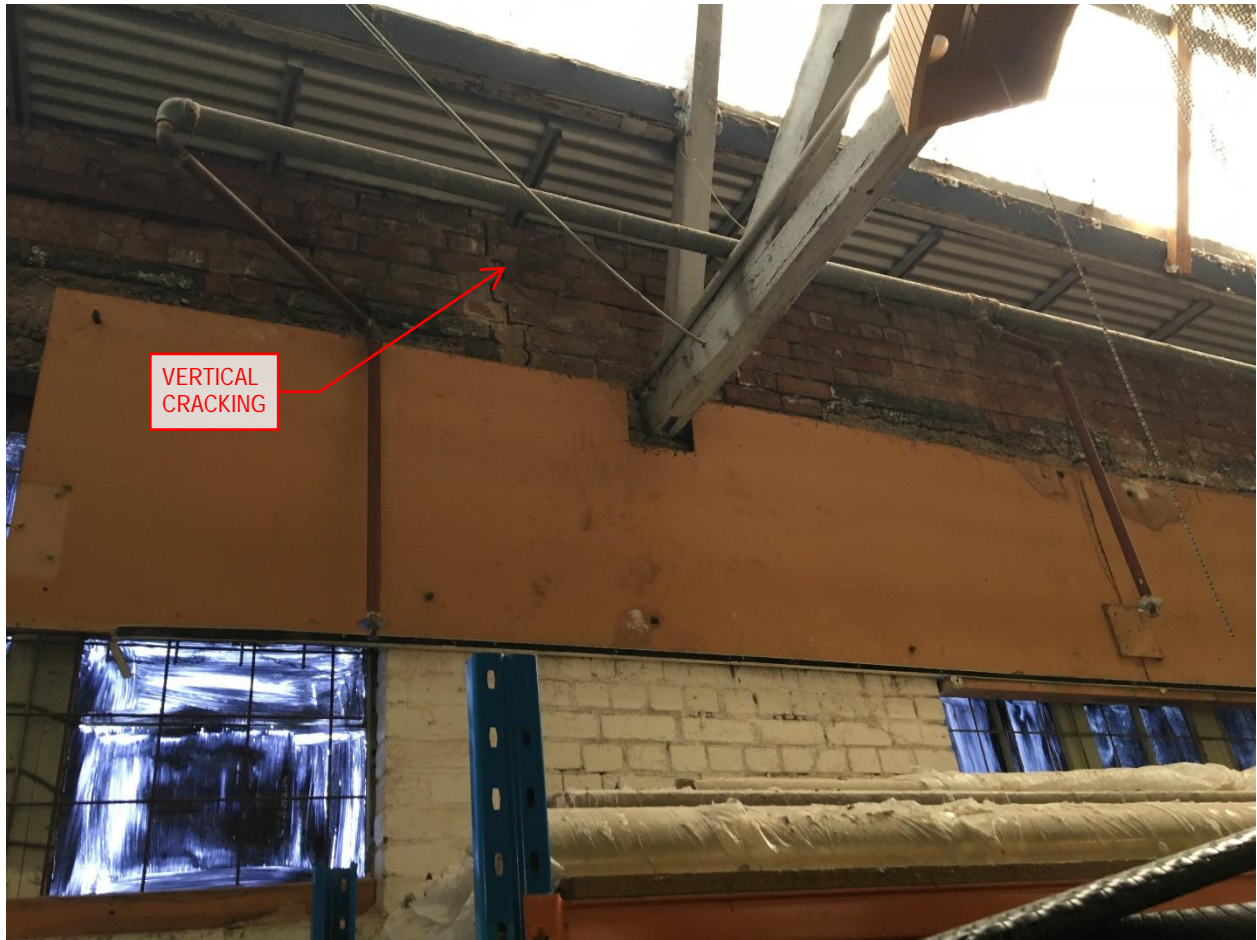
Image 2.5: Vertical cracking in masonry above lintels.
