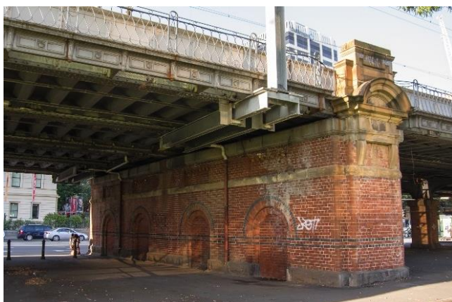
Figure 14. Brick structure with decorative sandstone end pediment (corner Market St). (Source: Context 2019)
