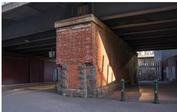
Figure 16. Bluestone foundation and quoining evident in one of the substructure. (Source: Context 2019)
