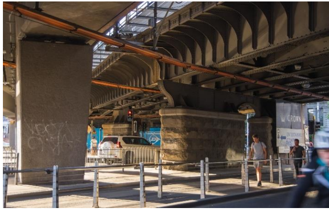
Figure 19. Spencer Street tram stop. Concrete piers dating from the 1970s, and the bluestone pier from 1917. (Source: Context 2019)
