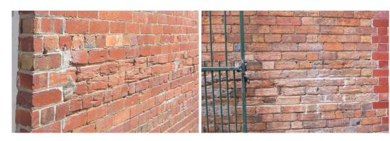
Figure 6. Vehicle marks on 27-29 Little Lonsdale (left) and a neighbouring building at 23-25 Little Lonsdale Street. (Source: Context 2018)
