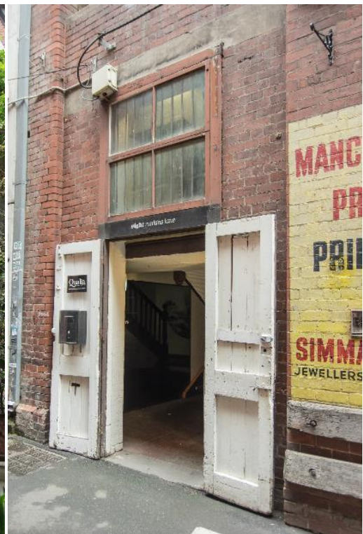
Figure 12. Example of intact openings and timber doors and windows at 8-14 Rankins Lane. (Source: Context, January 2020)
