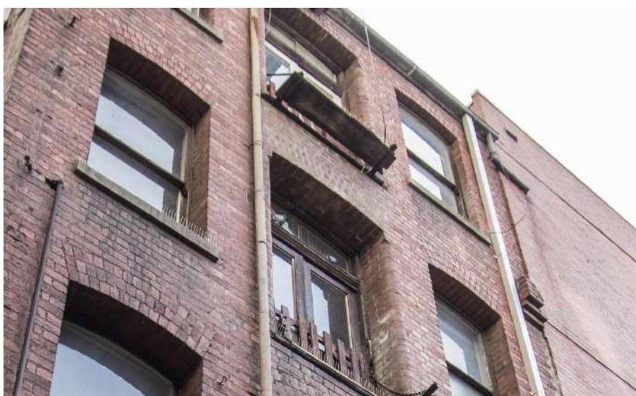
Figure 22. Note the remnant corbelled bracket on the northern (RHS) edge of the second floor of 3 Kirks Lane. (source: Context, January 2019)
