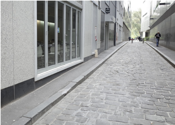
Existing heritage bluestone pitch paving
