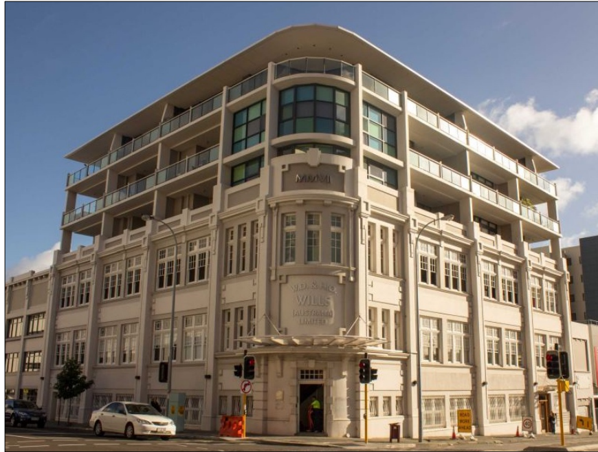
Figure 13 Former WD & HO Wills warehouse, Perth. Three additional levels were built above the heritage facade at minimal setback. The project was the recipient of the 2009 WA Heritage Council Award for Excellence in Adaptive Reuse.
