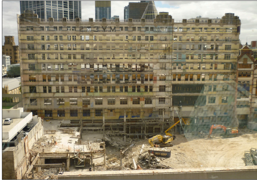
Figure 16 A 2012 photograph of the showing the demolition of the Myer Emporium with only the Lonsdale Street facade retained.
