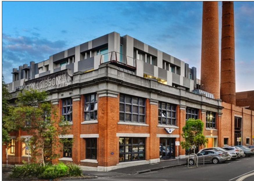
Figure 15 Rooftop additions at minimal setback from the façade of a former Foy & Gibson boiler house, Collingwood. The building is listed on the Victorian Heritage Register (VHR H755).
