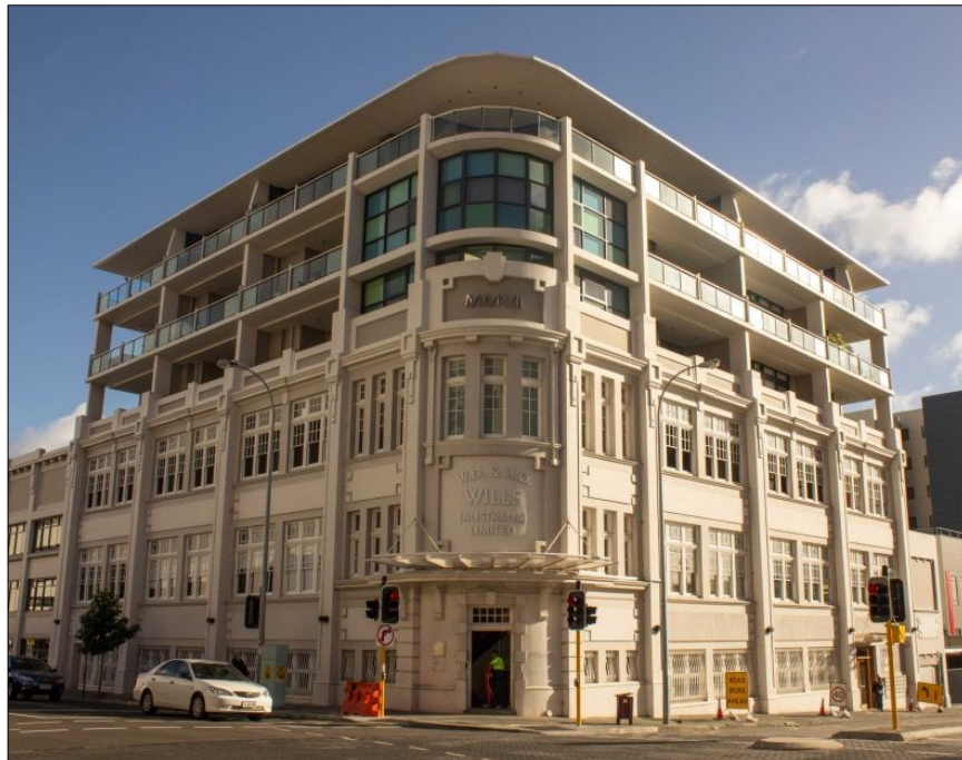
Figure 18 Former WD & HO Wills warehouse, Perth. Three additional levels were built above the heritage façade at minimal setback. The project was the recipient of the 2009 WA Heritage Council Award for Excellence in Adaptive Reuse.
