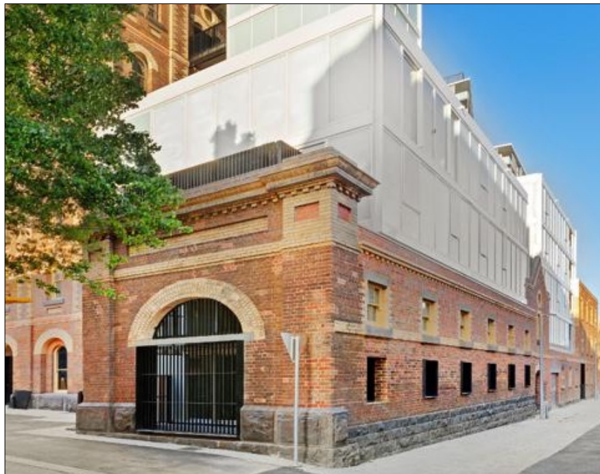
Figure 16 Part of the redeveloped former Yorkshire Brewery showing modern upper storey additions with a modest front setback and no setback to the side elevation of the retained heritage façade. The former Yorkshire Brewery is included on the Victorian Heritage Register (VHR H807).
