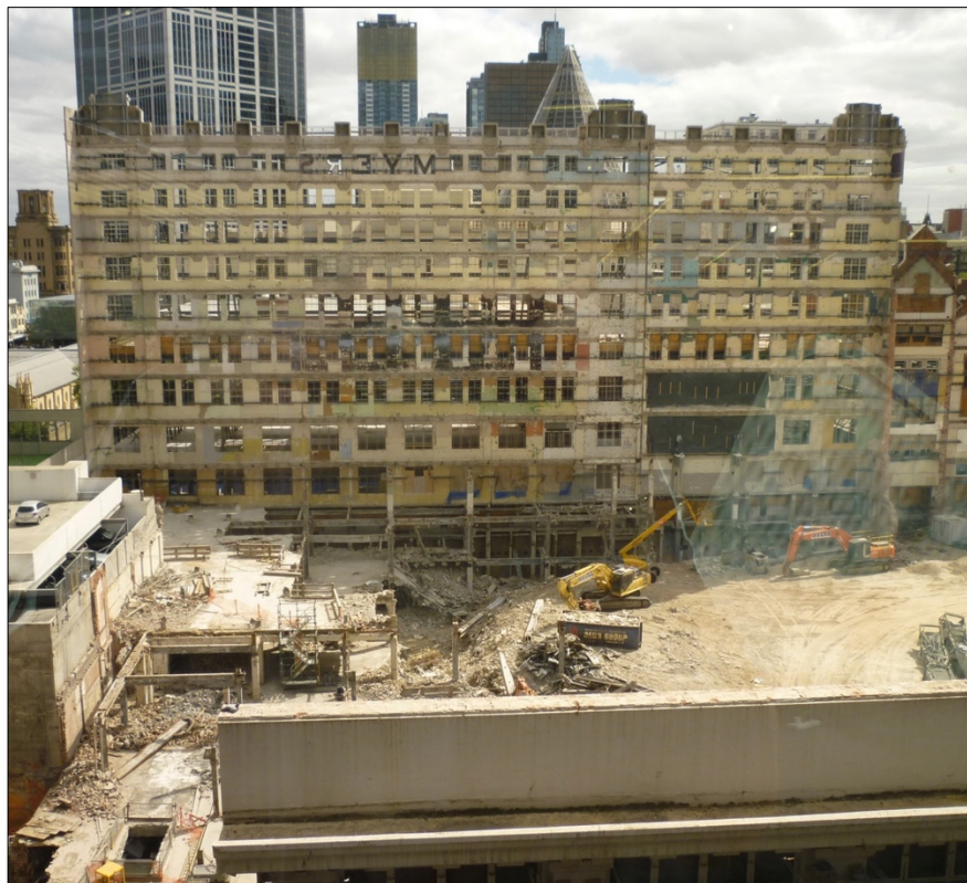
Figure 20 A 2012 photograph showing the demolition of the Myer Emporium in progress with only the Lonsdale Street facade retained.
